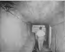
PROBABLY the only tunnel in regular use in Aruba has been closed. The tunnel, pictured above a few days before it was sealed, led from the head of the No. 1 Finger Pier to the old Plant Dispensary. It admitted non-employees, principally from visiting ships, to the enclosed dispensary area but not to the refinery proper. Opened about 1949, it was closed when the new Employee Medical Center went into operation.
